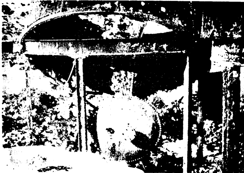
Figure 3-1 Rusting of abandoned steel tank.
