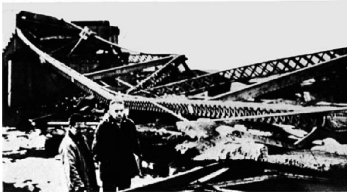
On December 15, 1967, the Silver Bridge connecting Ohio and West Virginia over the Ohio River collapsed, and 46 people lost their lives. The cause of the collapse was stress-corrosion cracking
