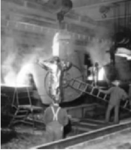
Figure 9: Steel-making machinery [wikipedia]
